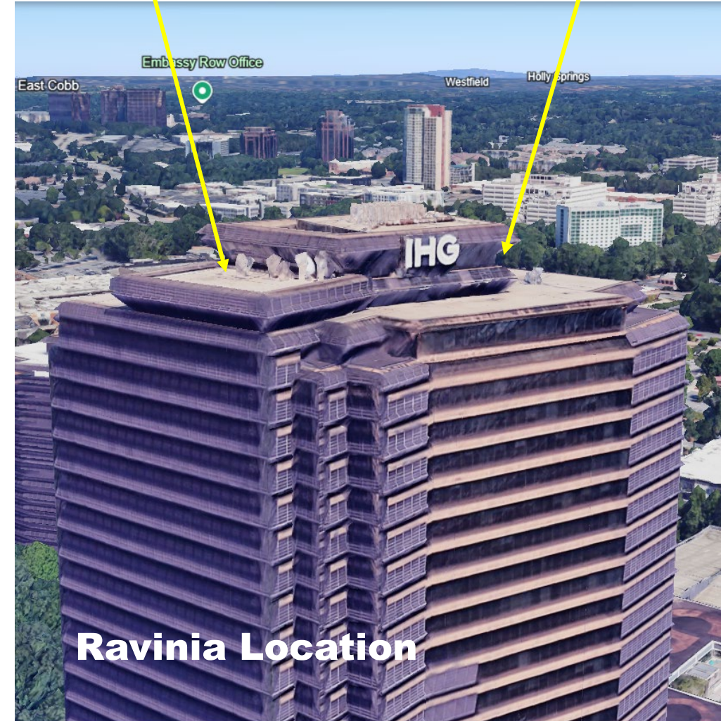
Dekalb County Network Room inside the Building
